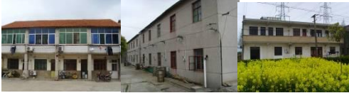
Figure 12. Two-storey joint uniform architectures
